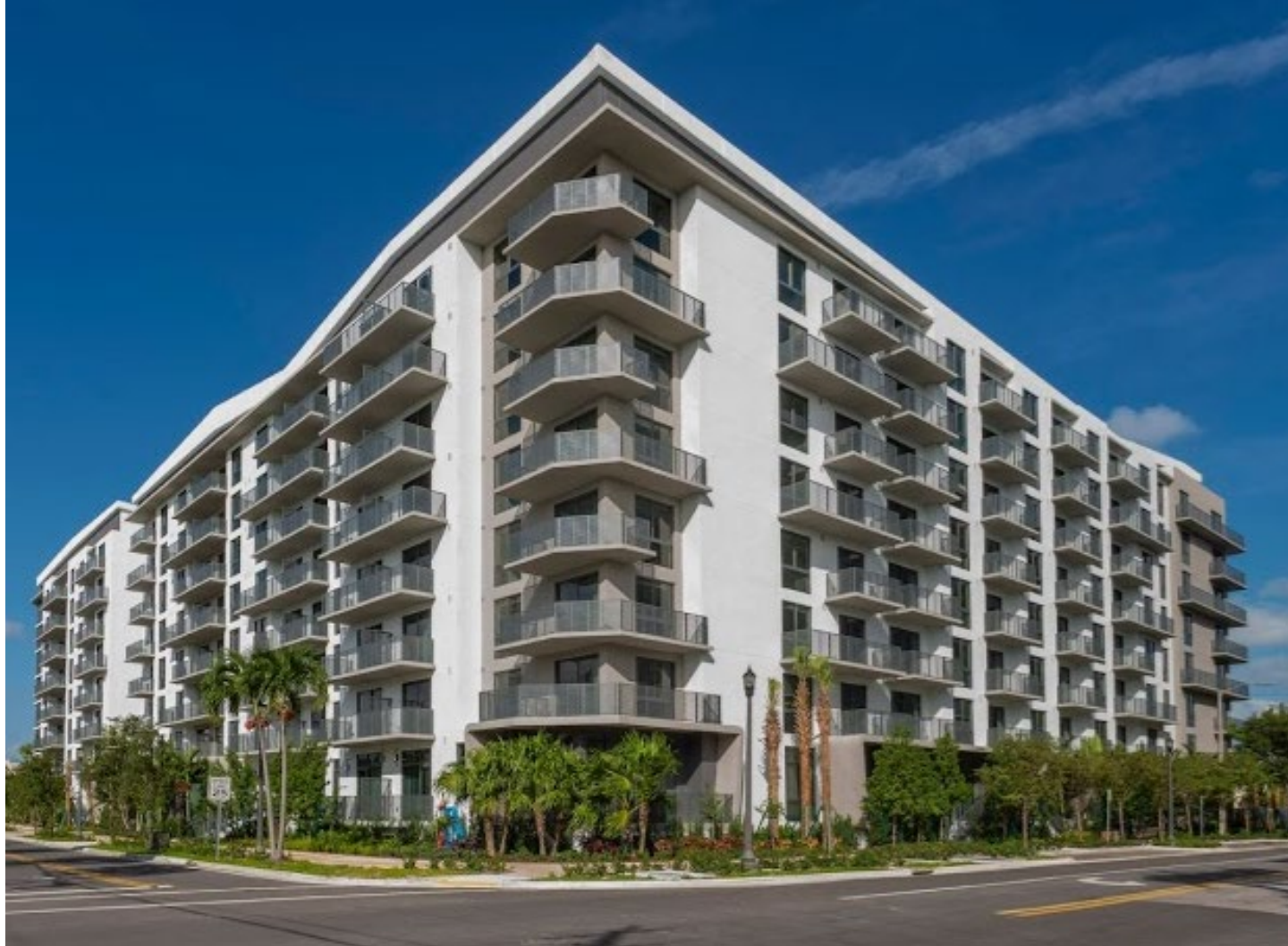
New Waterline Miami River Project located across the river at 1001 NW 7th Street
